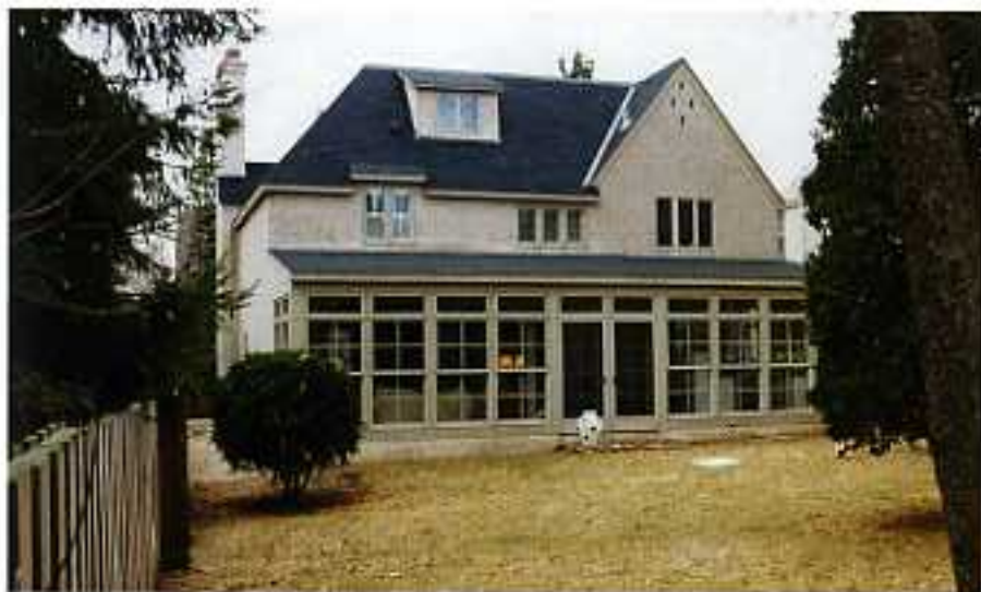
The preconstruction view shows a barren and open space lacking both spatial articulation and privacy.
